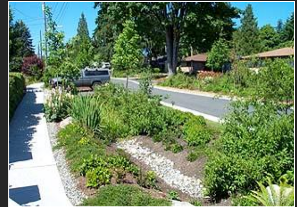
GI for Stormwater Management (City of Philadelphia)
